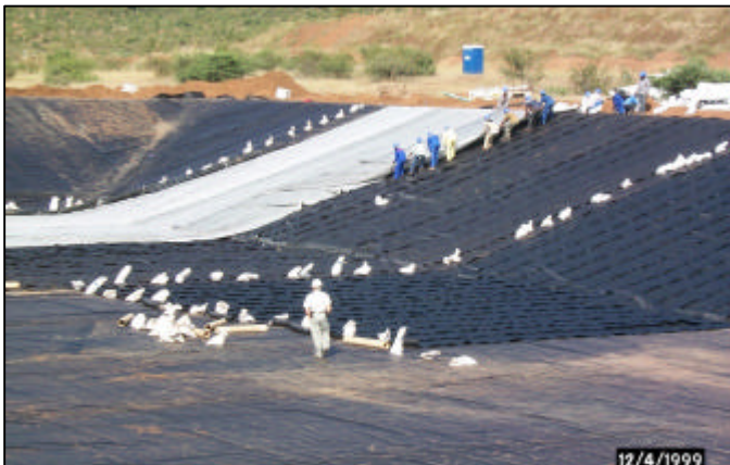
Hi-drain Installation at Platkop
